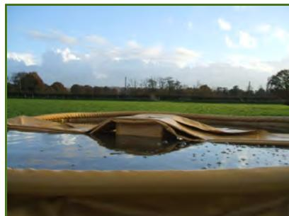
Pull the cover over the tank evenly until central, with the float section positioned in contact with the water.
