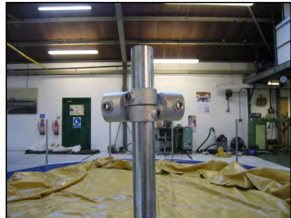
5. Connect all the legs together with the lower horizontal poles at the base of the leg. We recommend that the horizontal poles should be approximately 120mm above ground level.
