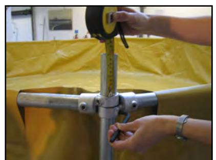
Ensure that the swivel pole connectors at the top are set at the correct height and angle. The correct height is 100mm from the top, as illustrated above. The correct angle is set by eye using the edge of the liner base as a guide.
