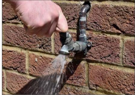
**2** Open the tap and leave water running for at least **one minute** before taking a sample. **DO NOT** adjust the flow of water during this time. This ensures that any deposits in the pipes are washed out and the water sample is representative of the water in the supply pipes.
