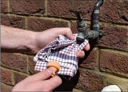
**1** Remove any attachments from the tap; e.g. nozzles, pipes, etc. and wipe around the tap with a clean cloth.
