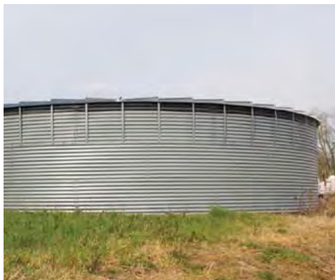
A new large above ground store
