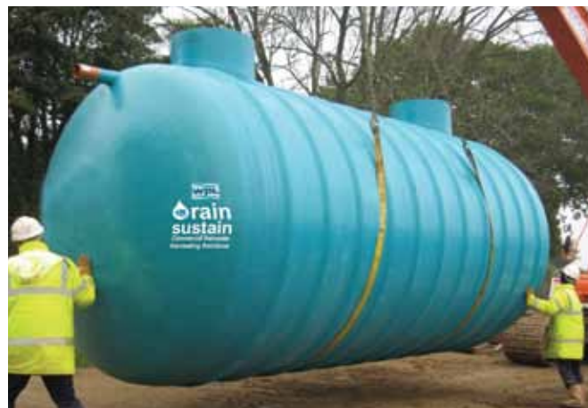
Figure 5 → Examples of underground storage tanks
