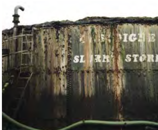
You can reduce the size of the slurry store that you need if you divert clean roofwater away from the store
