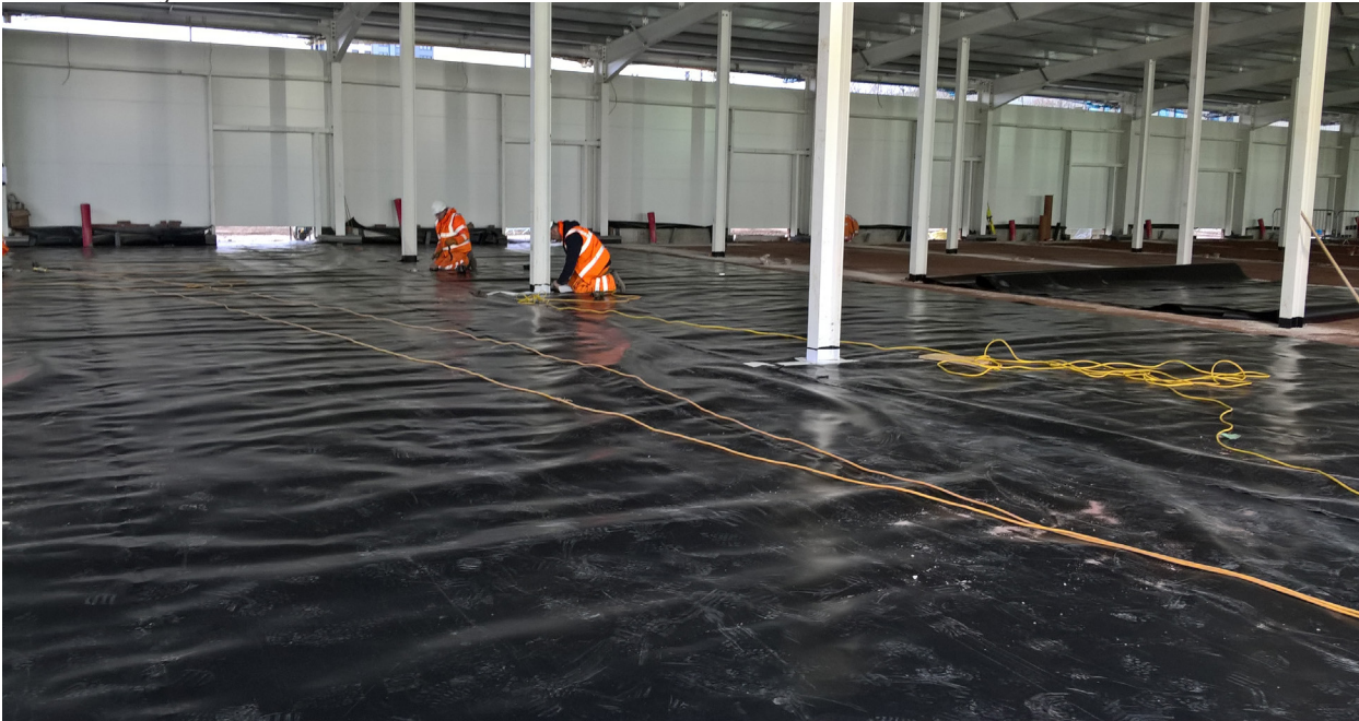
Gas membrane installation for a retail outlet in Liverpool
